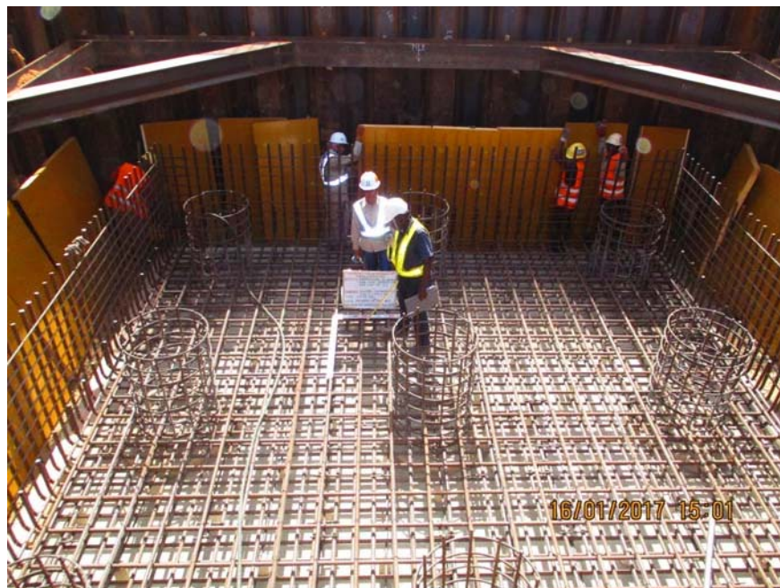
Bottom Re-bars for Pile Cap
