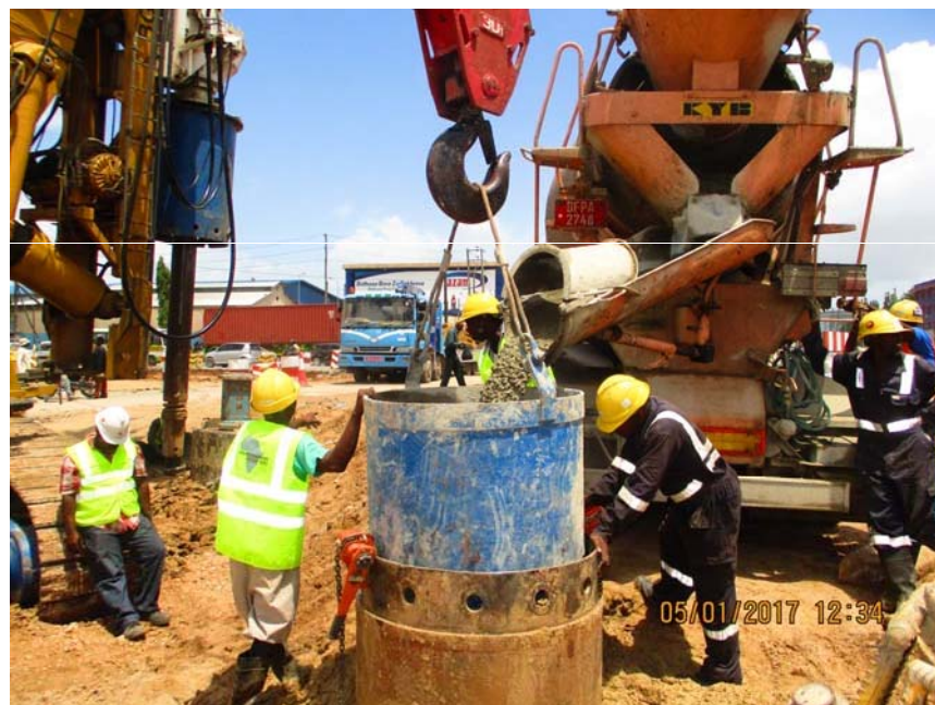
Concreting with Tremie Pipe
