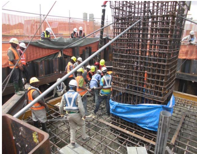
Concreting Pile Cap
