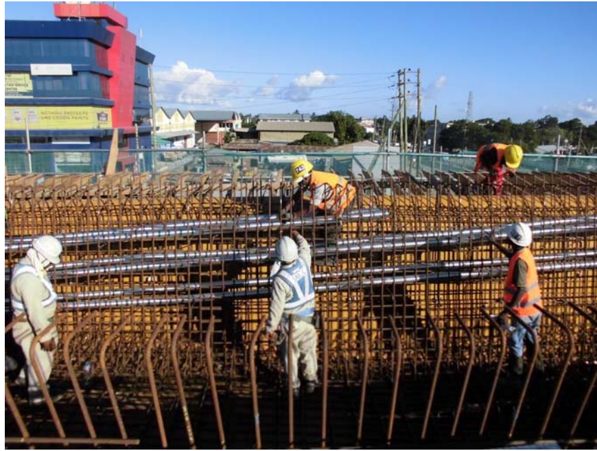
Reinforcement Bar and Pre-stressed Concrete (PC) Cable Work for Hollow Slab
