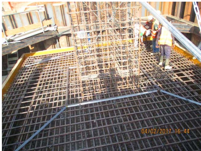
Ready for Pile Cap Concreting
