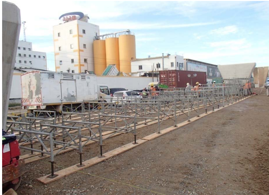
Scaffolding Work for Hollow Slab
