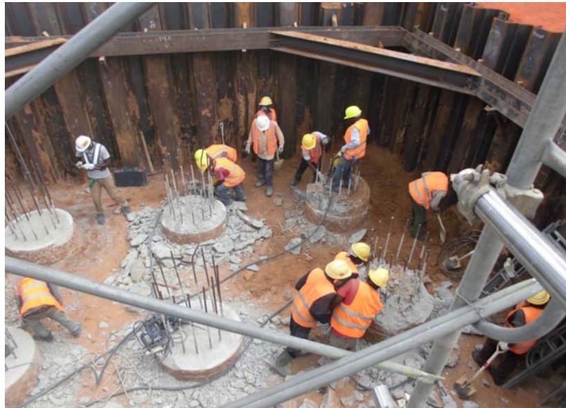
Pile Head Treatment after Excavation
