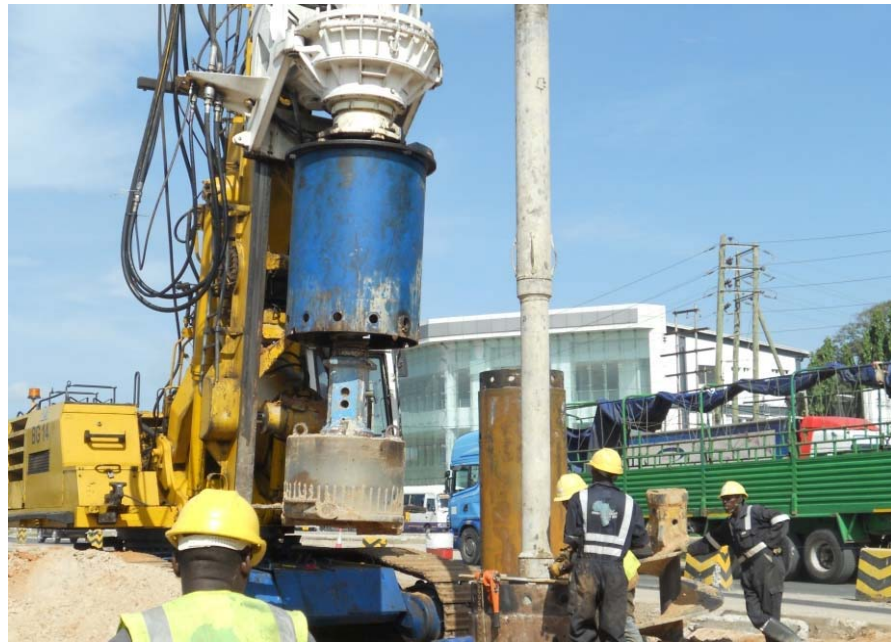
Installation of Tremie Pipe
