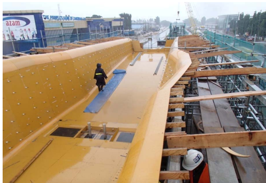
Formwork for Box Girder
