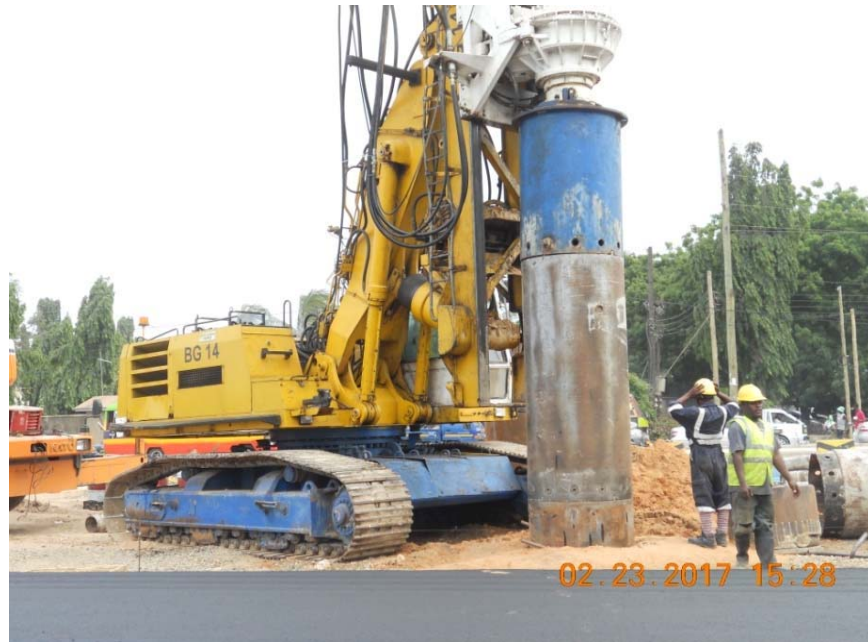
Extraction of Casing Pipe
