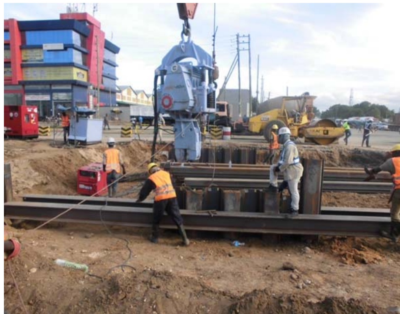
Driving Steel Sheet Piles for Cofferdam
