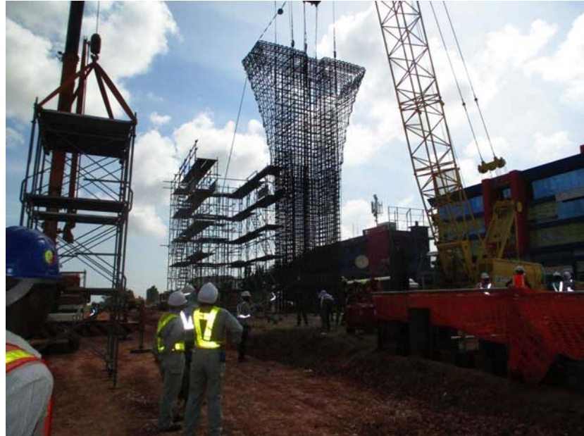
Installation of Pre-fabricated Re-bars for Pier Column
