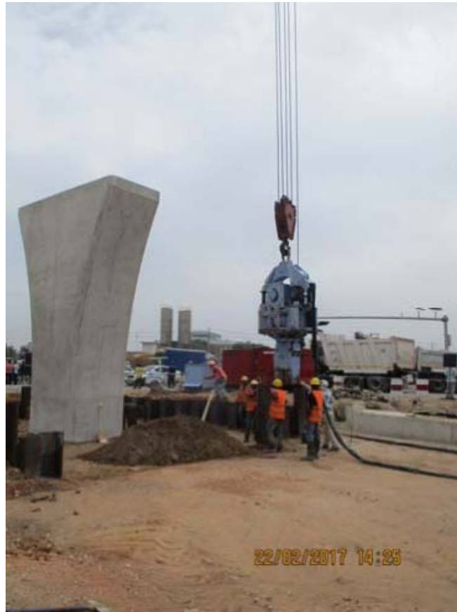
Back Filling & Removing Sheet Piles
