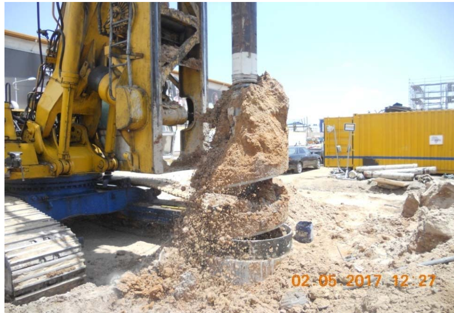
Excavation for Bore Hole
