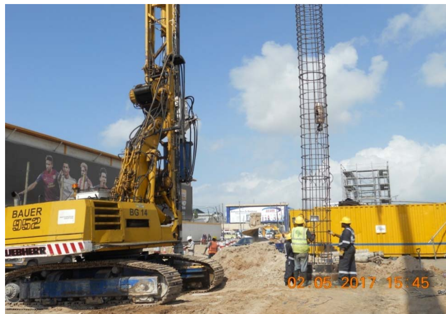
Installation of Re-bar Cage
