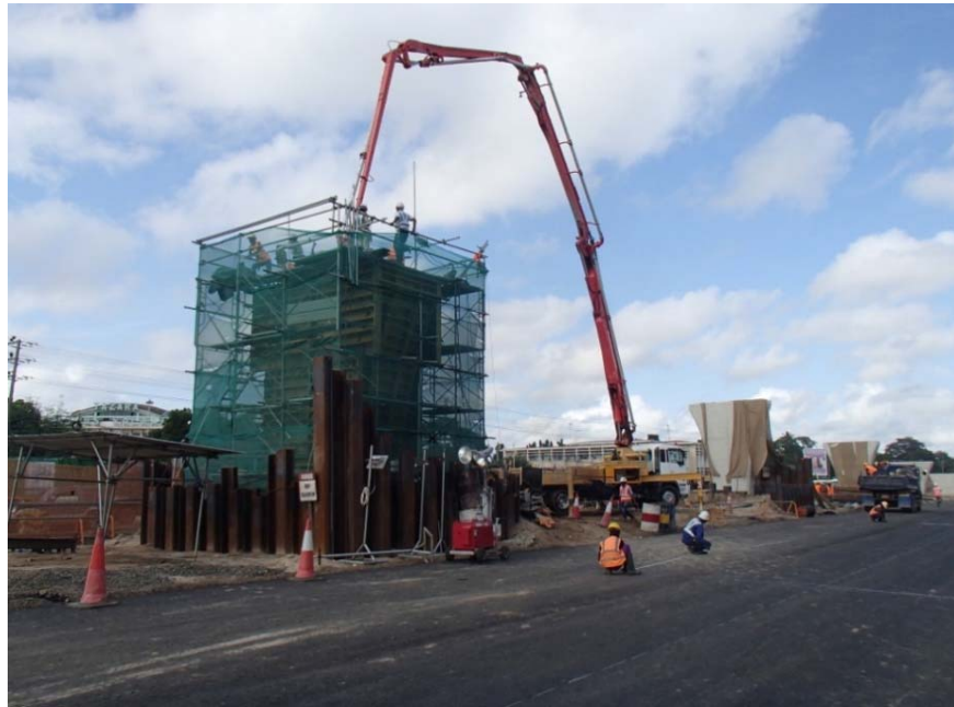
Concreting Pier Column [2nd Lift]
