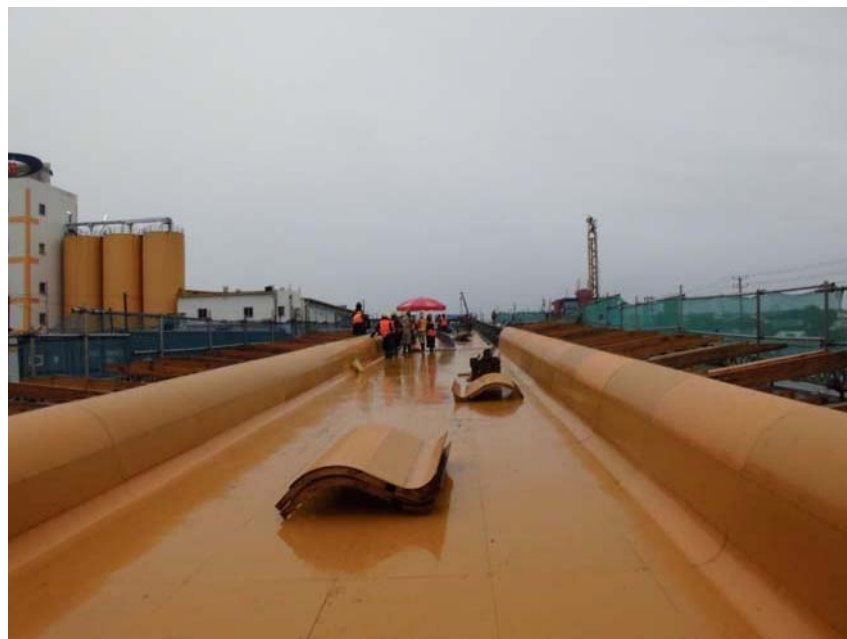
Formwork for Hollow Slab
