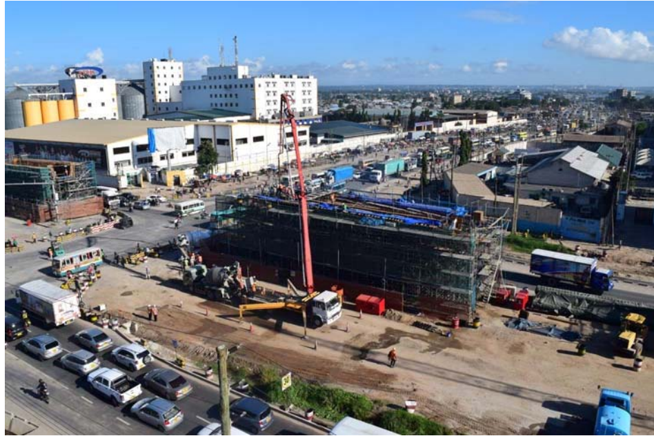
Concreting Works for Box Girder
