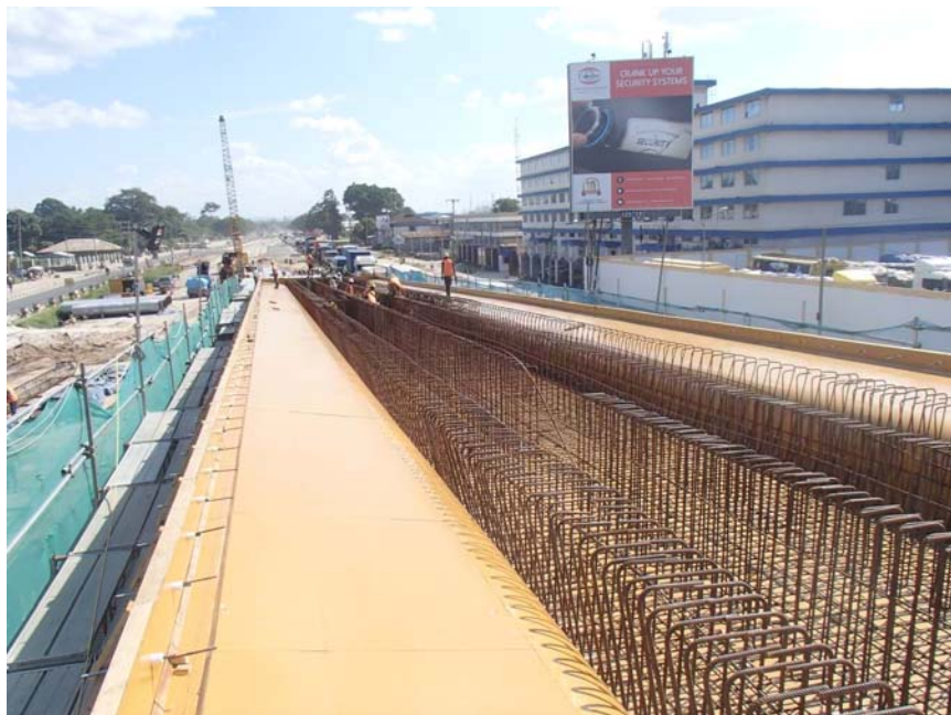
Reinforcement Bars Fixing Works for Hollow Slab
