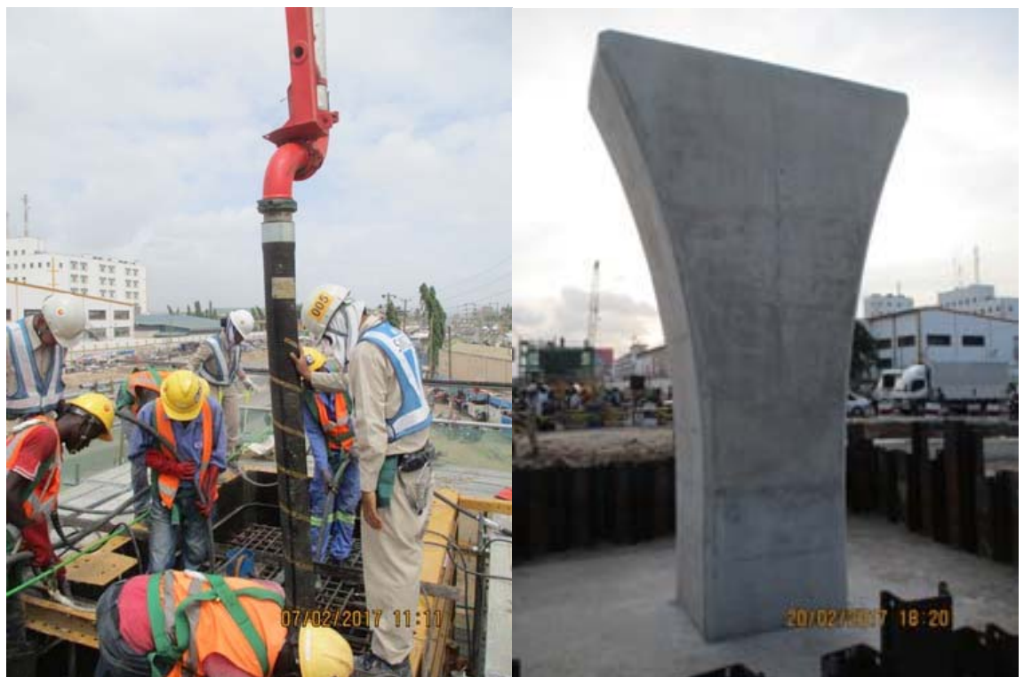
Concreting Pier Column [2nd Lift]
