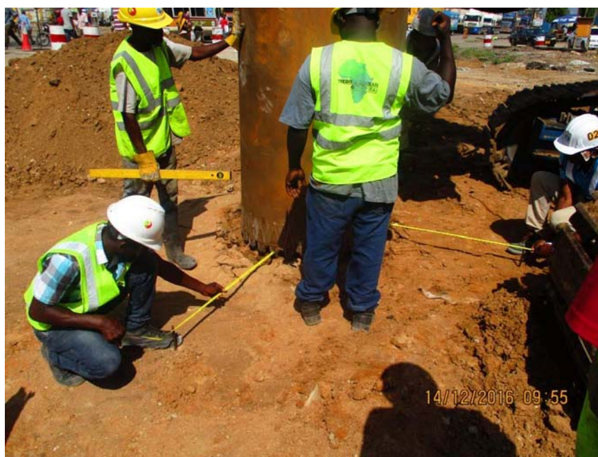
Taking Position of Bored Pile Casing
