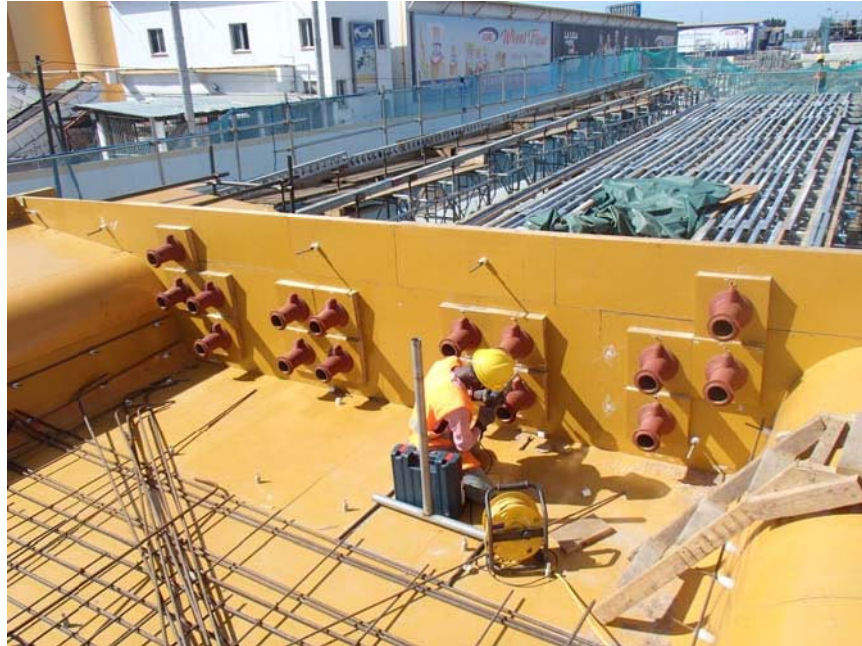
Formwork of Pre-stressed Concrete (PC) Anchor for Hollow Slab
